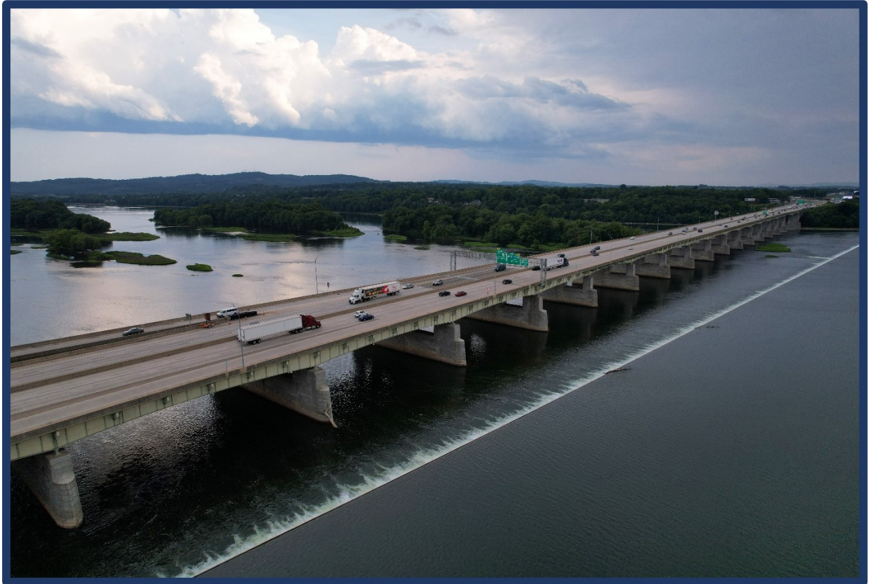
I-83 South Bridge in Dauphin County
