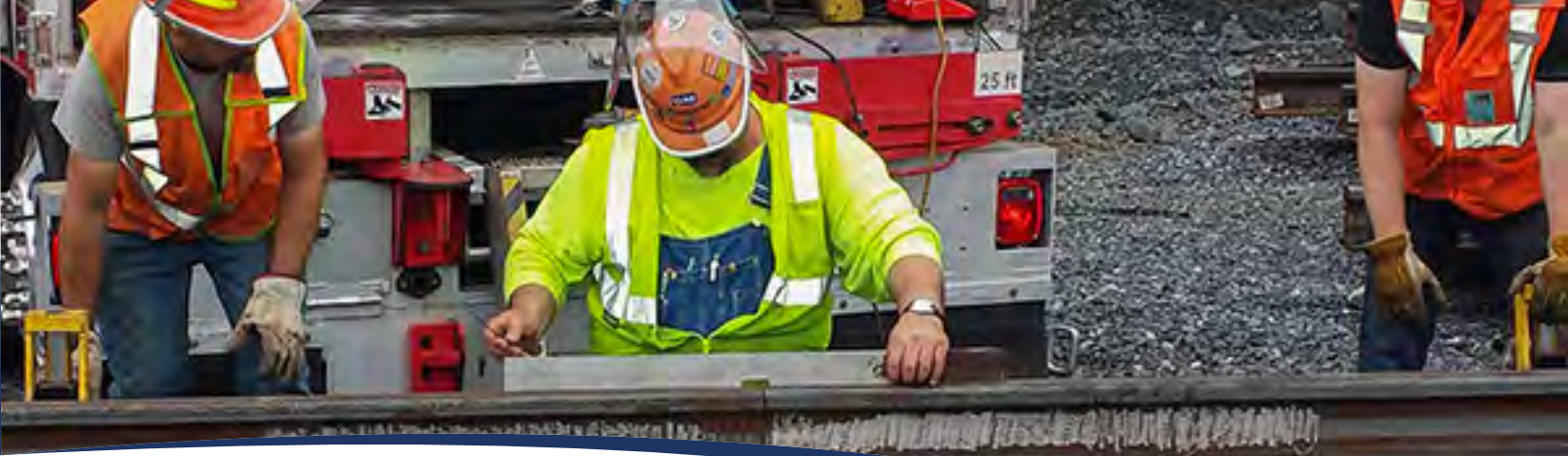
Welding foreman aligning rail ends at Middletown Station, Dauphin County Courtesy of PennDOT
