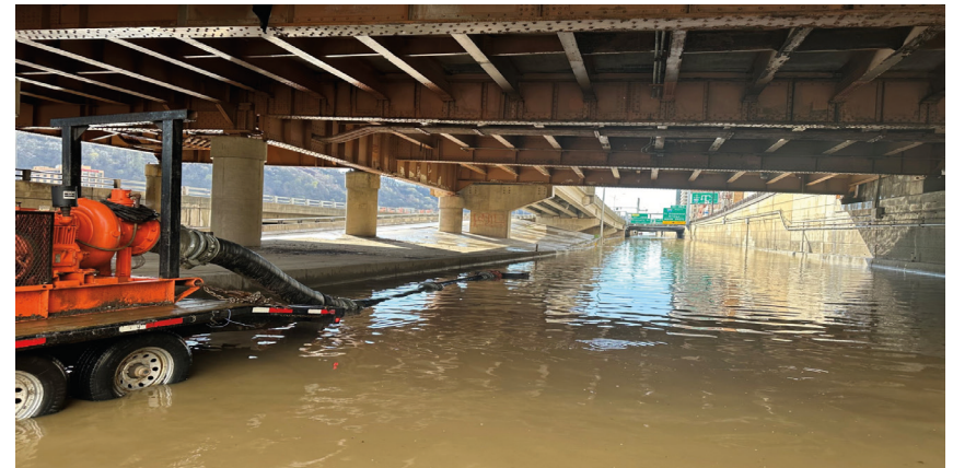
Dewatering pump for I-376 (Parkway East) flooding event cleanup.
