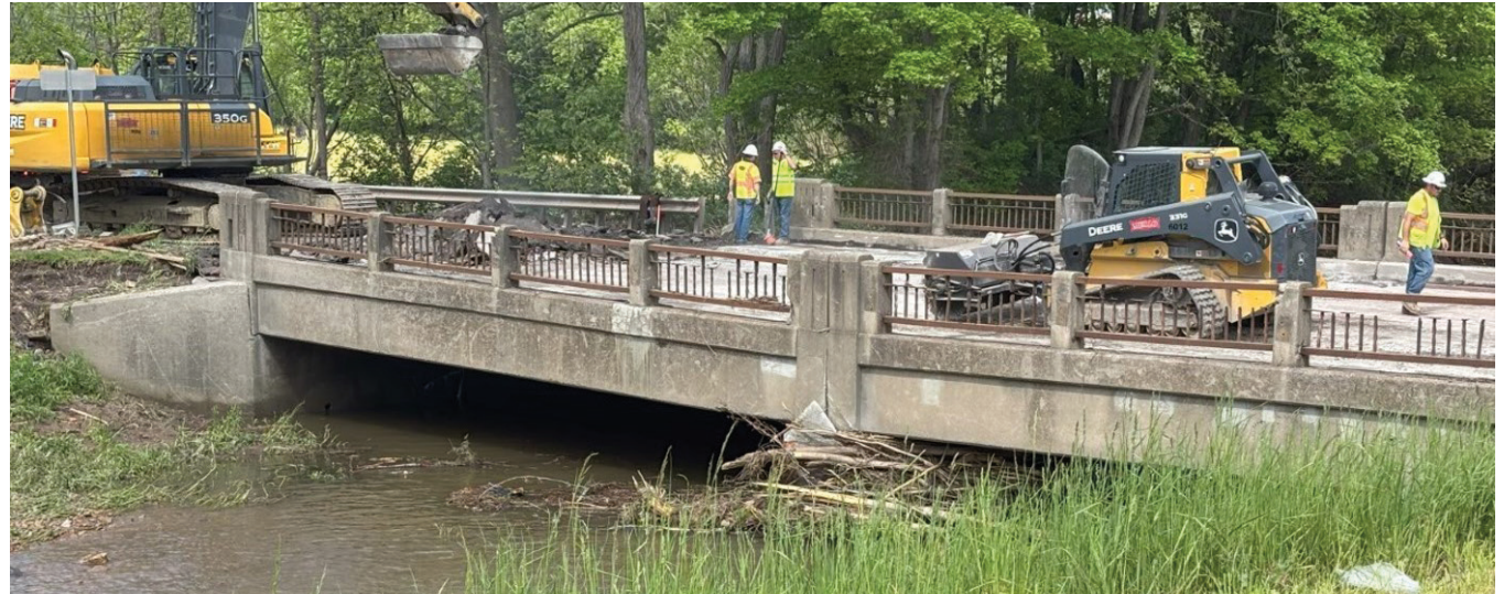
On May 16, 2025, two days after the bridge was closed, demolition began on the 102-year-old bridge.
