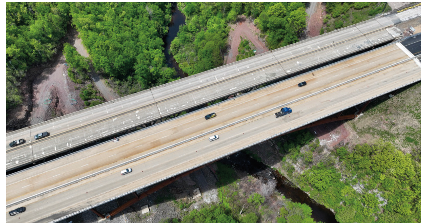
Drone image of the newly completed Hawk Falls Bridge in Carbon County, Pa. May 26, 2026.
