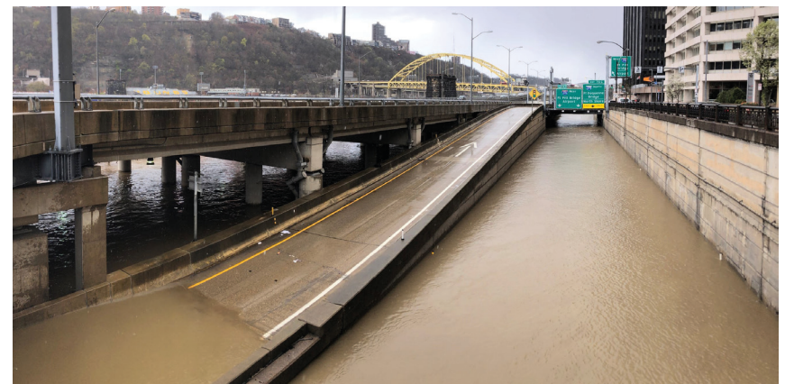
Monongahela River flooding event on I-376 (Parkway East).
