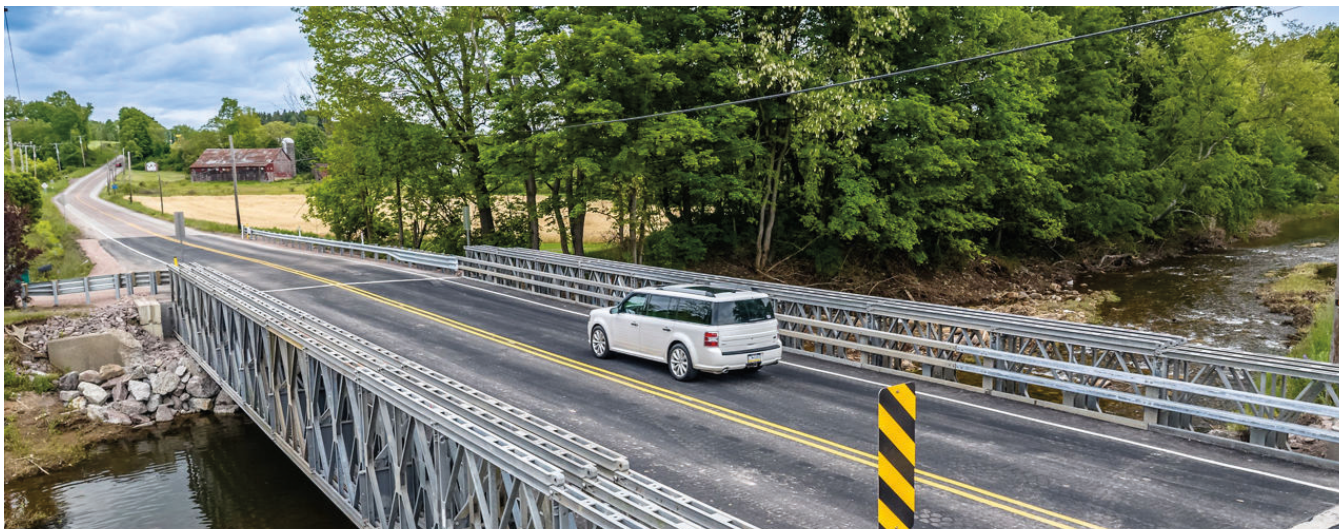
On May 24, 2025, just 10 days after the Boynton Bridge failure, U.S. 219 reopened to traffic in time for the Memorial Day weekend. Image Credit: ©Acrow Bridge 2025.
