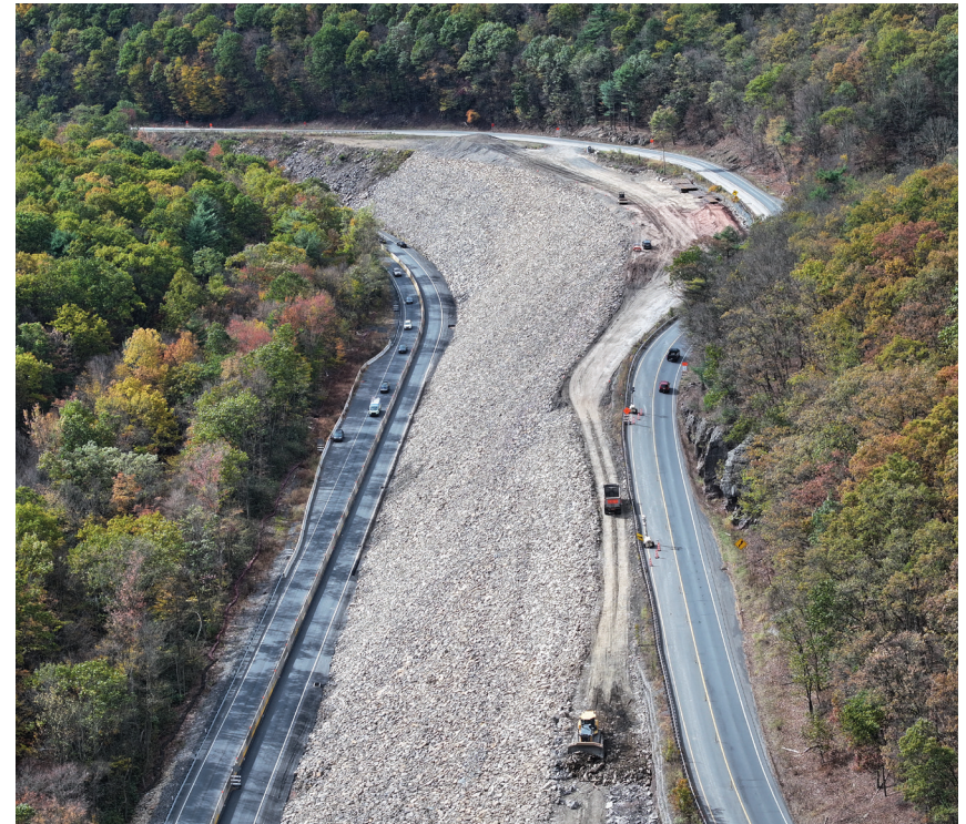
Route 61 widening and curve realignment construction.
