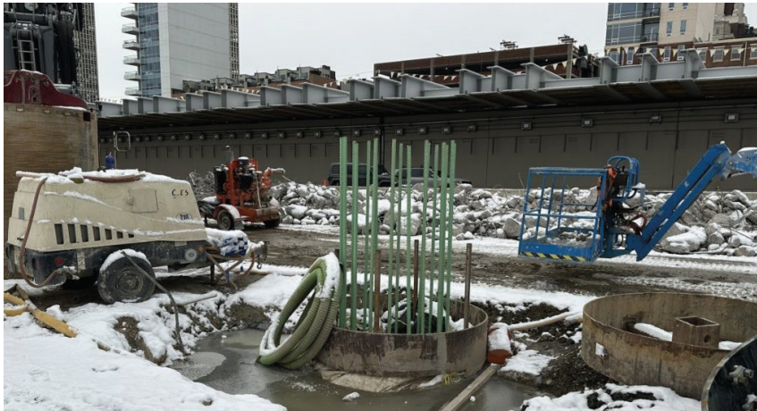
I-95 CAP Project abutment and support pier construction.
