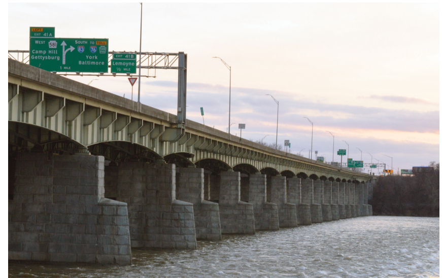
Interstate 83 John Harris Memorial (South) Bridge.
