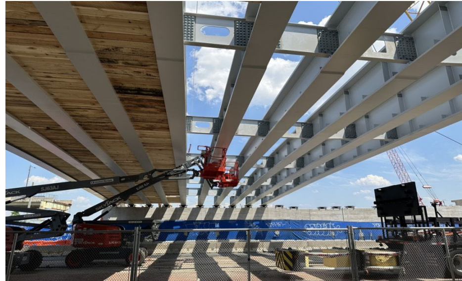
(18 deck beams placed in late May.)
