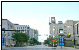
12 th Street Corridor Signal Improvements
