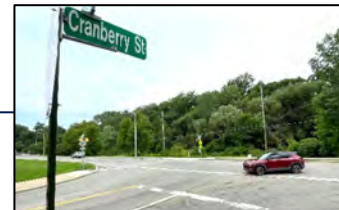
Cranberry Street Signal Installation
